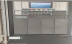
Fire Alarm Control Panel
